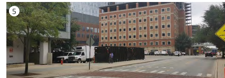
Service Corridor – 12 th Avenue
