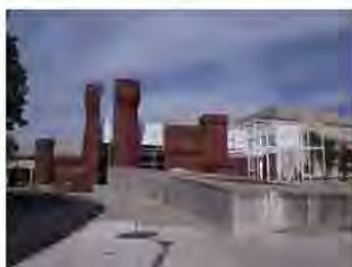
Figure 1.2.2 The Wexner Center for the Arts
